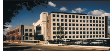
Figure 1. The new Central Laboratory of the Virginia Division of Forensic Science is located in downtown Richmond, Virginia.
